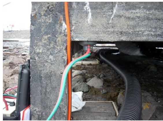
Fig. 8 – Test on underside of concrete beam
