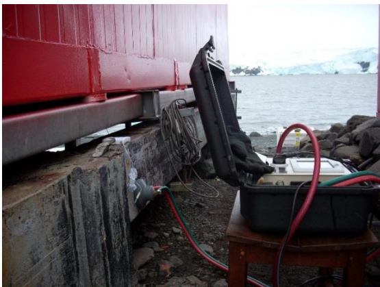
Fig. 7 – Test on vertical coated surface
